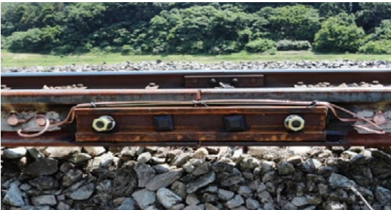
The copper exothermic welding for railway application
