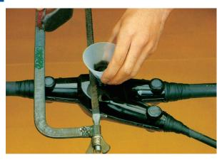
① After the resin has hardened - this should take 60 to 80 minutes - cut the funnels away with metal cutting saw.
